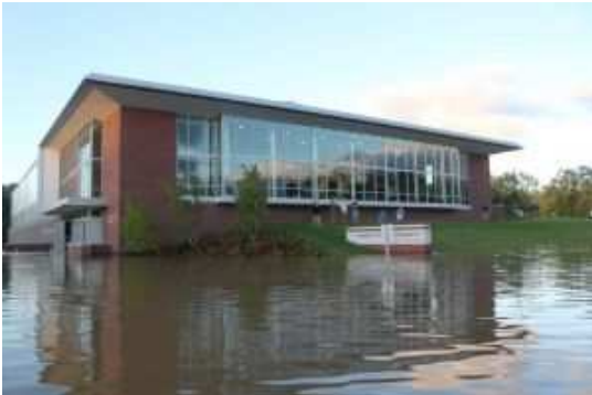
Flooding from the Pemigewasset River encroached on the campus of Plymouth State U.
